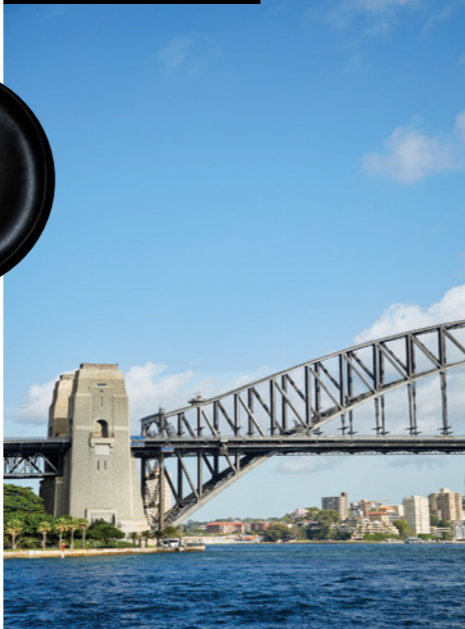
SYDNEY HARBOUR BRIDGE
